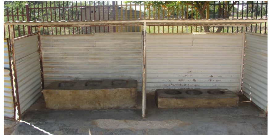
Figure 1: Toilets used by the children at Thusanang Centre
