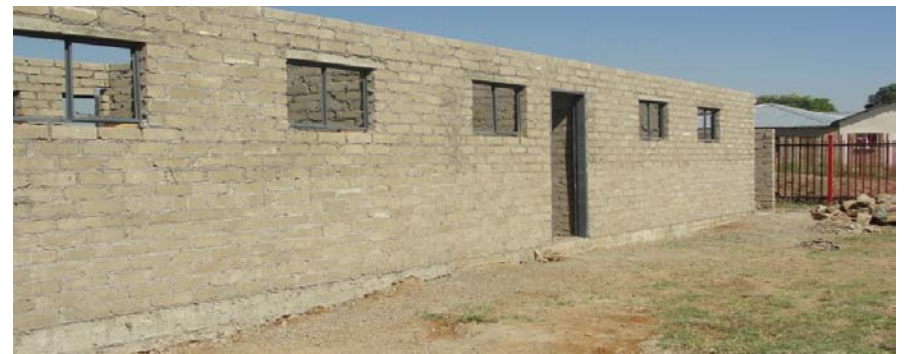
Figure 5: The new toilets built with the NDA grant funds.
